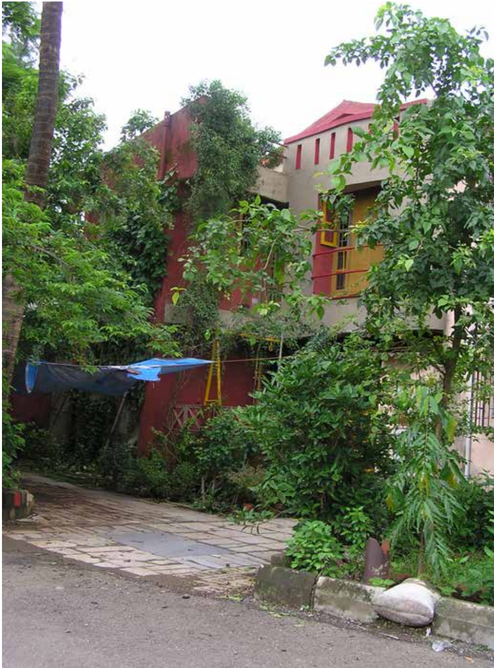
Figure 5: Residual space encroached upon by a resident. Photo credit: author
